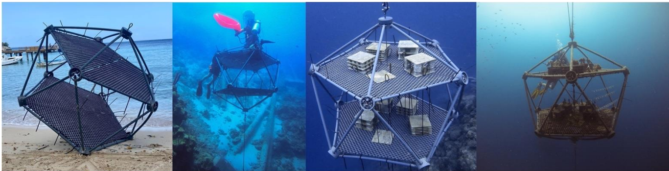
Figure S26: Two-Platform Arks. (Left) Two-Platform Ark prior to beach deployment. (Middle left) Two-Platform Ark shortly after attaching to the mooring system. Lift bags at the top of the Arks are used to provide temporary buoyancy prior to the addition of mooring buoys. (Middle right) Two-Platform Ark after the addition of limestone ARMS. (Right) Two-Platform Ark system after 1 year of deployment.
