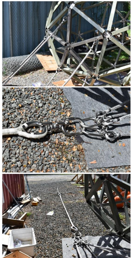
Figure S17: Ark Mooring system. (Left) Diagram of Ark mooring system. (Top right) Bottom of Coral Ark structure showing 5-point mooring bridle (3/4" Dyneema lines) connected to the 5 padeyes at the base of the Ark. (Mid right) The lower portion of the Ark mooring bridle, showing 3 of the Dyneema mooring bridle lines connected to the left link, and 2 of the Dyneema mooring bridle lines connected to the right link, at the top of the stainless Masterlink using 1/2" stainless shackles. Also shown is the stainless swivel connecting the bottom of the stainless Masterlink to the top of the 1" nylon downline. (Bottom right) The 1" nylon downline connects the mooring bridle to a chain anchor bridle, consisting of 3 lengths of chain that meet at a single galvanized pear-shaped link and are each attached to their own sand anchor eye at the opposite end using 3/8" galvanized shackles.
