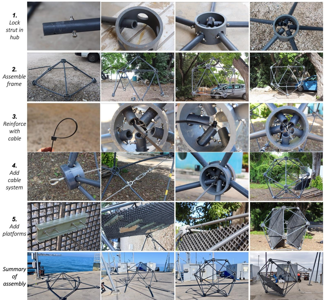
Figure S25: Assembly of Two-Platform Ark framework. Struts are inserted into hubs and locked into place via bolts and locknuts, and then a stainless-steel wire rope is passed through the finished structure to increase the strength. Two platforms are then added, bisecting the Ark horizontally.
